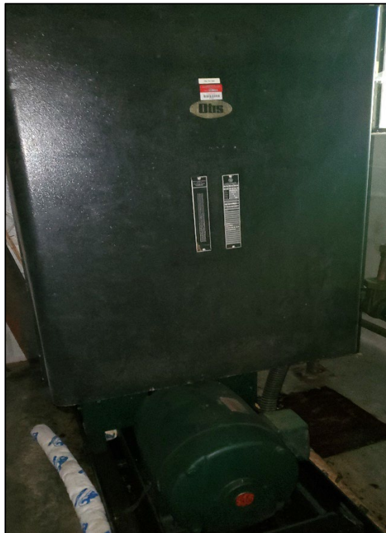
Photograph 14: View of hydraulic oil reservoir (elevator).
