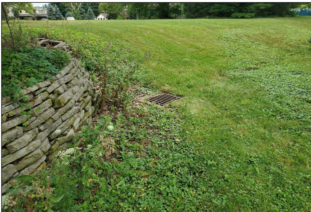
Photograph 11: View of a storm sewer catch basin (typical).
