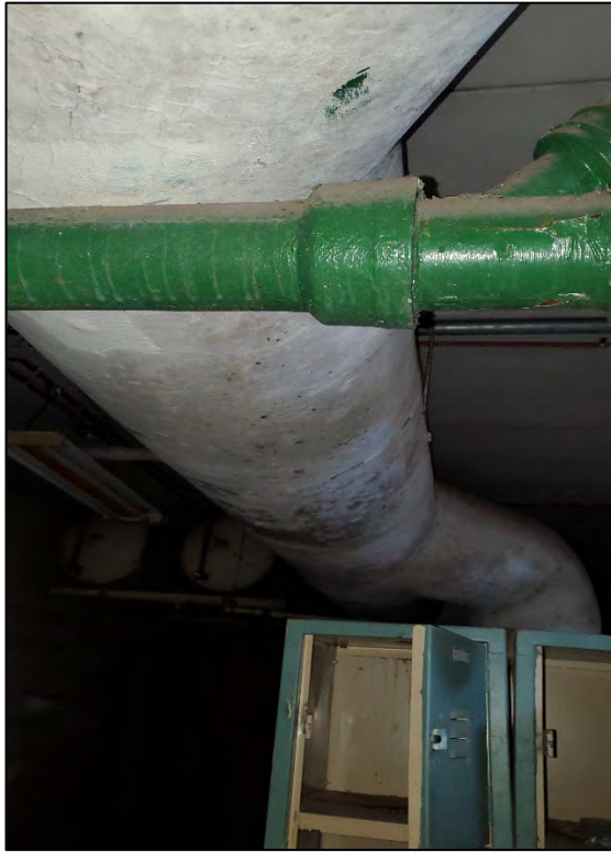
Photograph 15: View of ACM on the first floor of the building.
