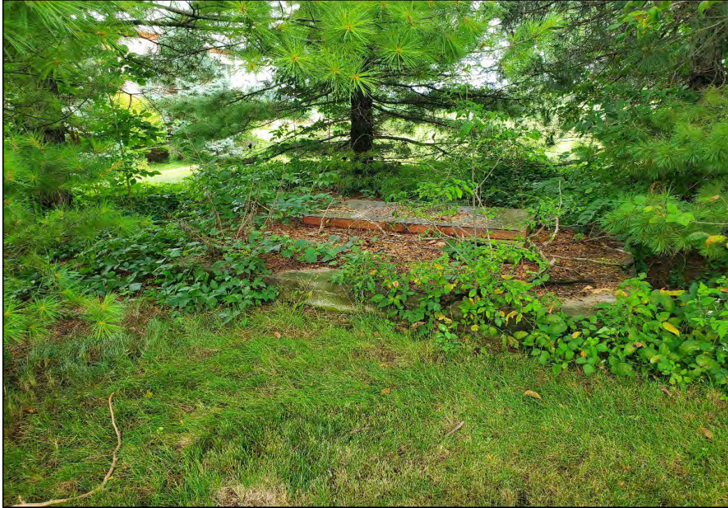
Photograph 13: View of the utility vault located south of the building..
