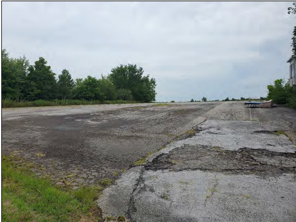
Photograph 8: View of the north parking area, looking east.
