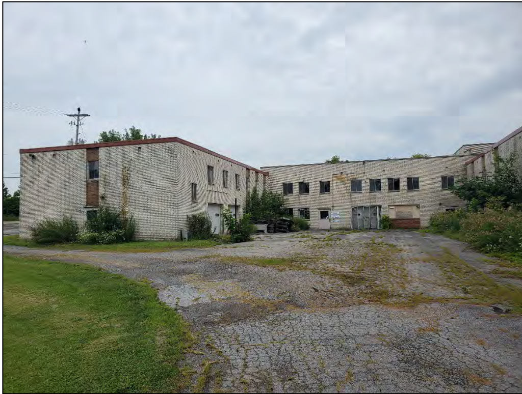
Photograph 9: View of asphalt area on the west side of the building.
