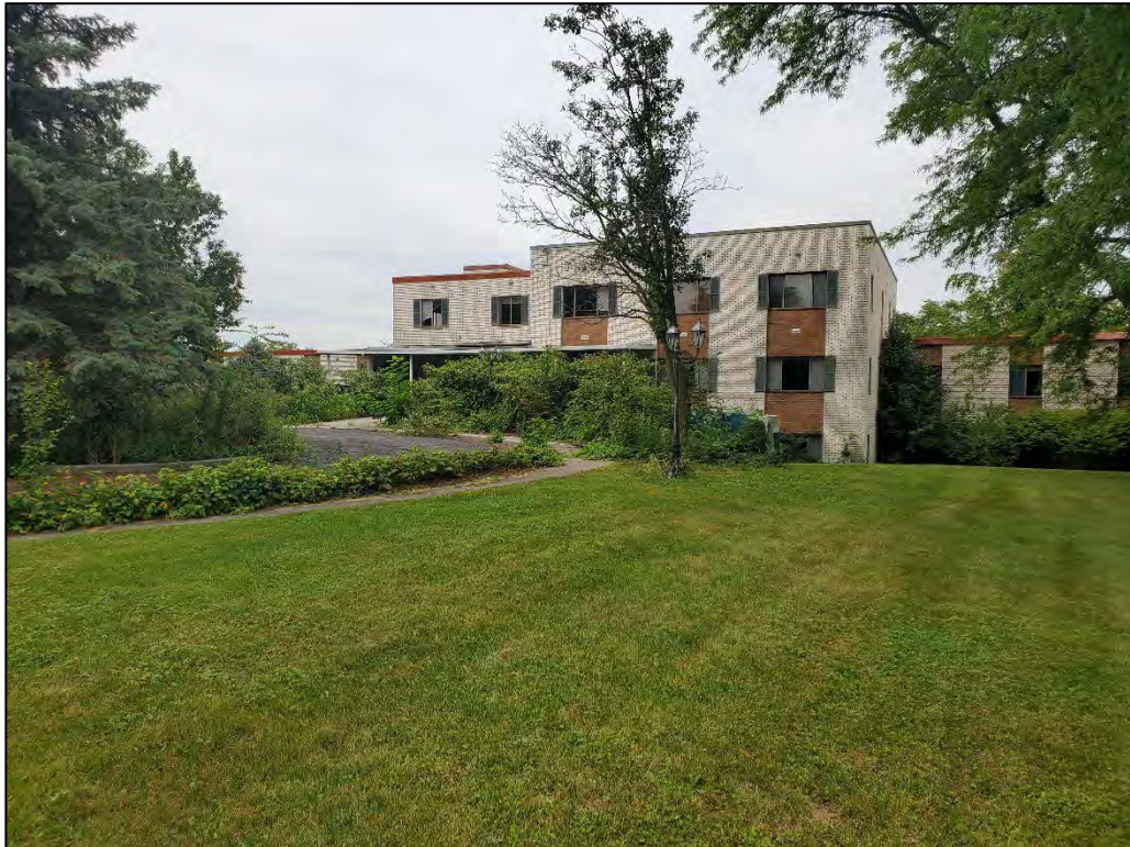
Photograph 4: View of the south façade of the building, looking north.
