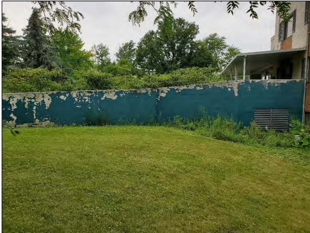
Photograph 2: View of the wing wall at the main building entrance.
