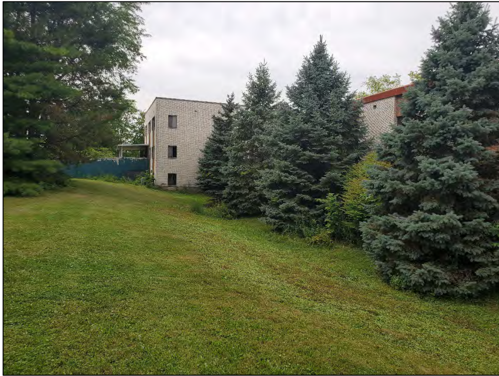
Photograph 1: View of the slope at the front of the building, looking west.
