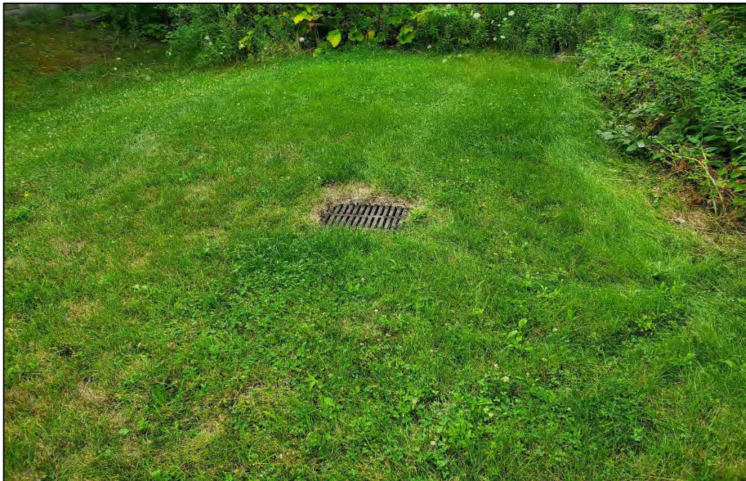
Photograph 11: View of a storm sewer catch basin (typical).
