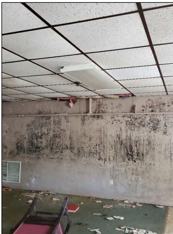
Photograph 18: View of a typical light fixture.
